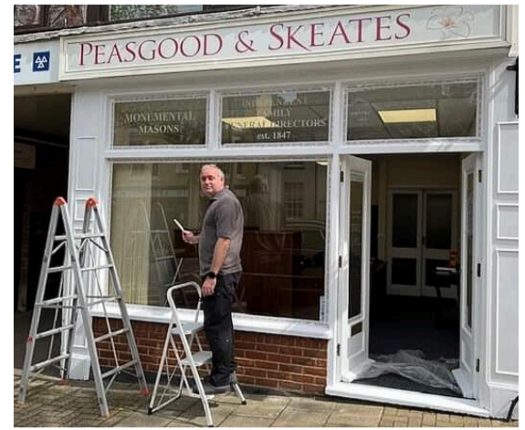
Neil Rogerson painting the new facade
